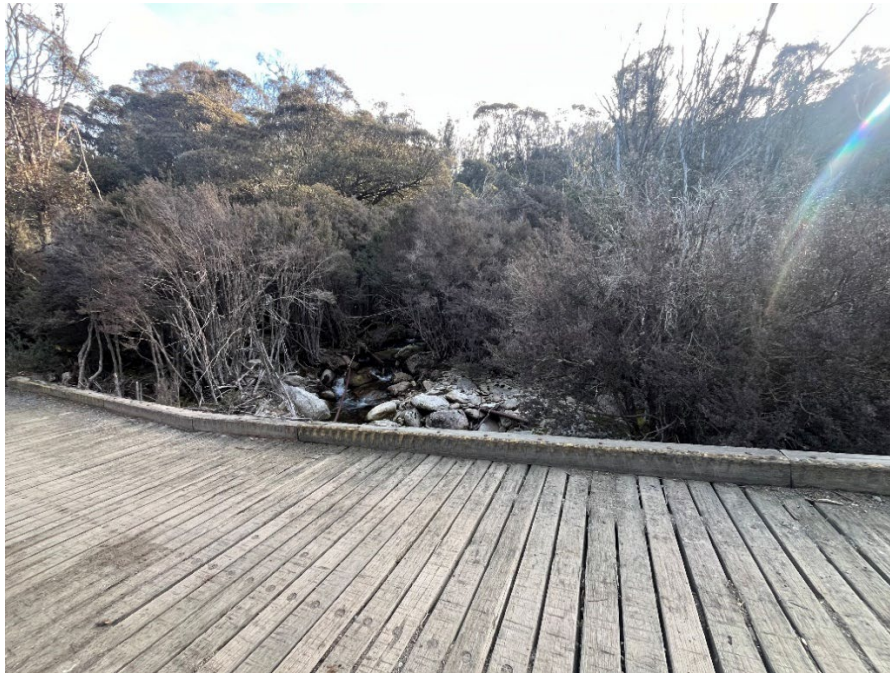
Figure 4: Reference point 1 facing upstream
